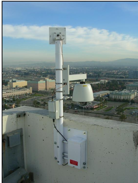
Figure 4. Wireless CCTV installation.
